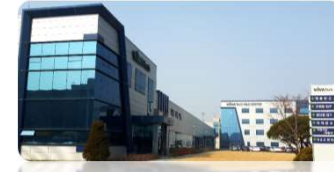
Energy Storage Device Leading Company
